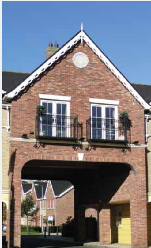
Extra heavy duty flat parabolic arch lintel
