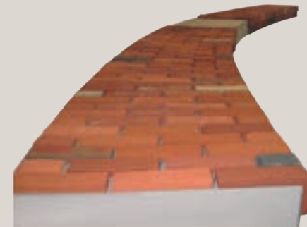
9m span arch Brick Feature Lintel provided to Tesco Central Offices, London.
