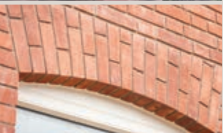
36 Cheswick Place, Birmingham
